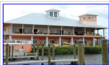
Laishley Crab House under construction.
